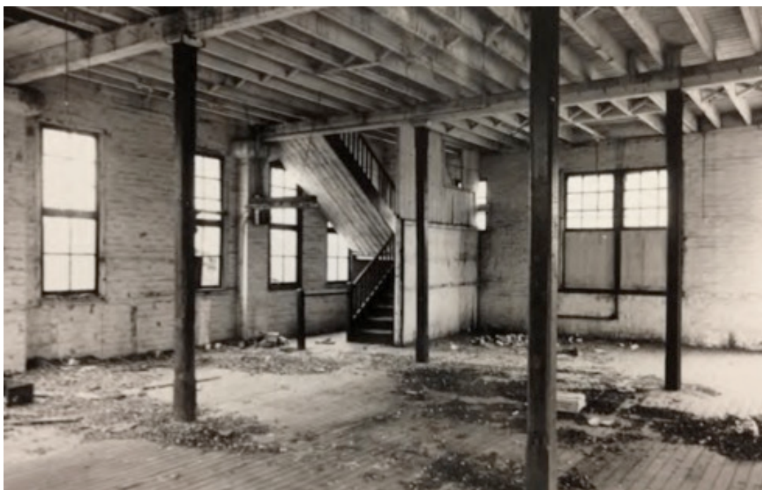
FIGURE 16: Interior view of the first floor of the factory in 1982, prior to renovation works. This photograph shows the original timber stair, now removed. Source: Waverley Local Studies Collection.
